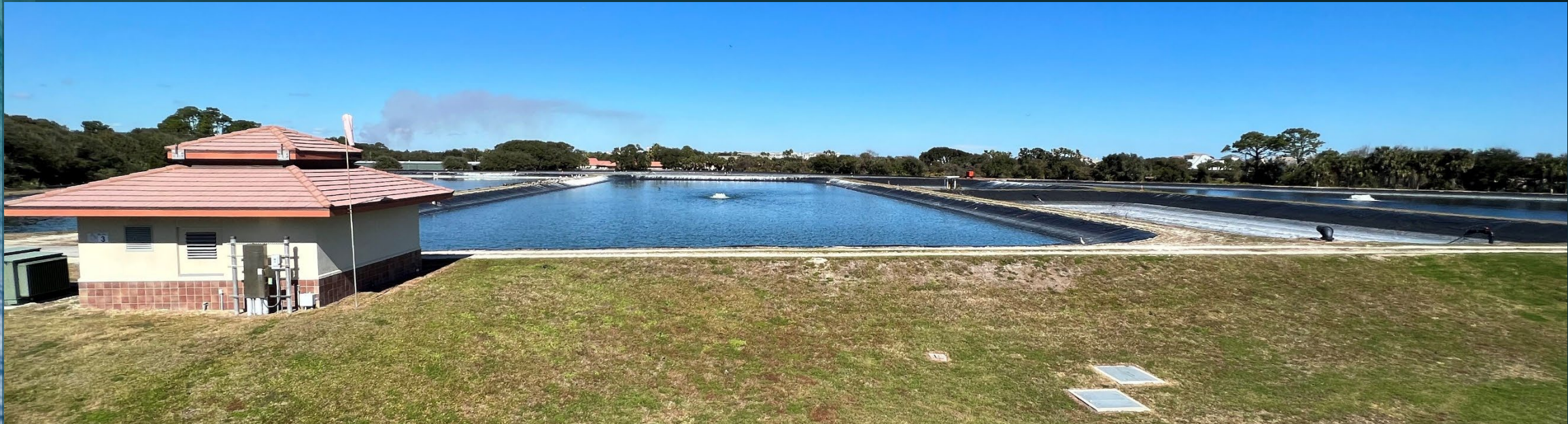
Reclaimed Pump Station and 18 Million Gallons of Reclaimed Ponds
