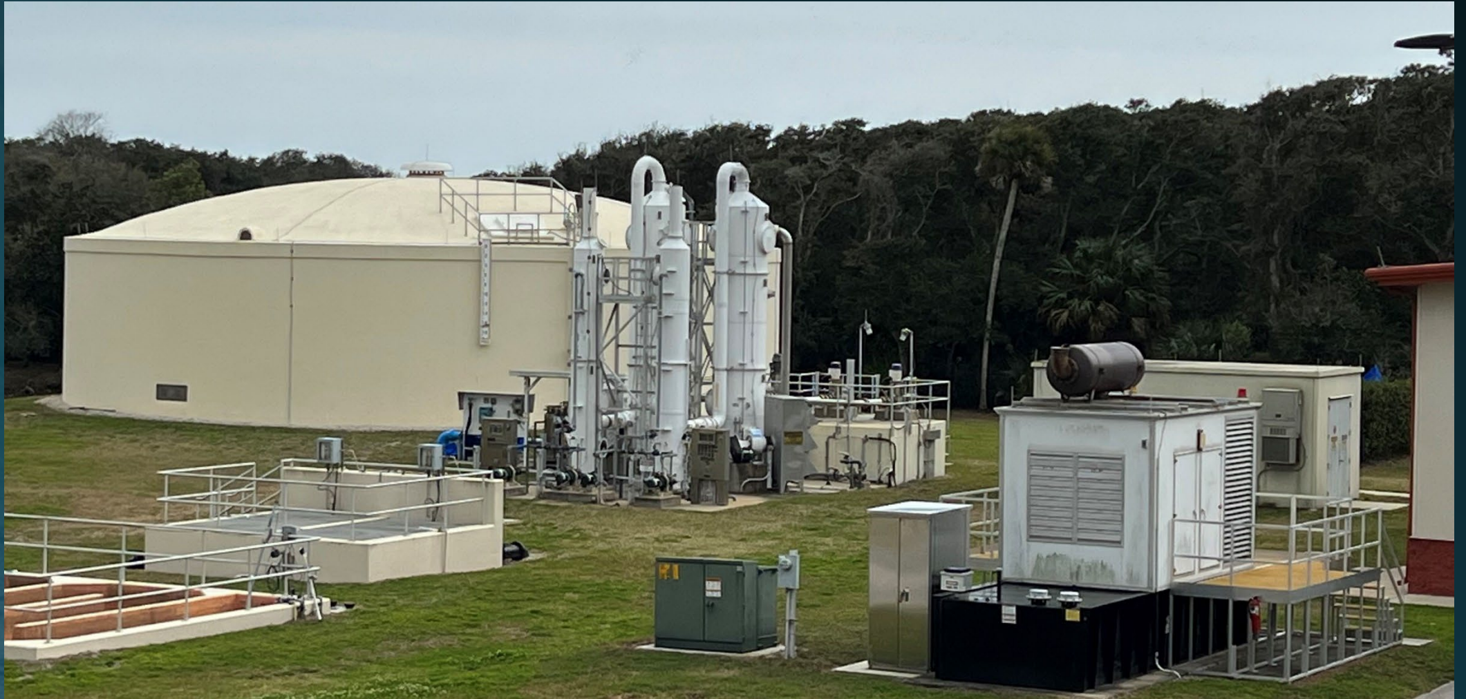
Potable Water Treatment Plant
