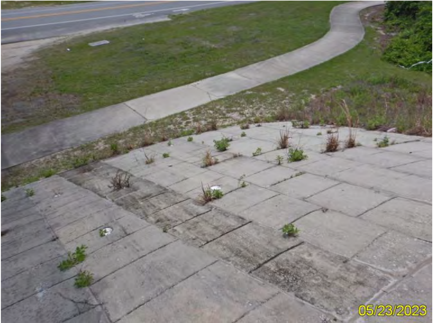
Photo 24 - Element 8394 R/Conc Abut Slope Protection
