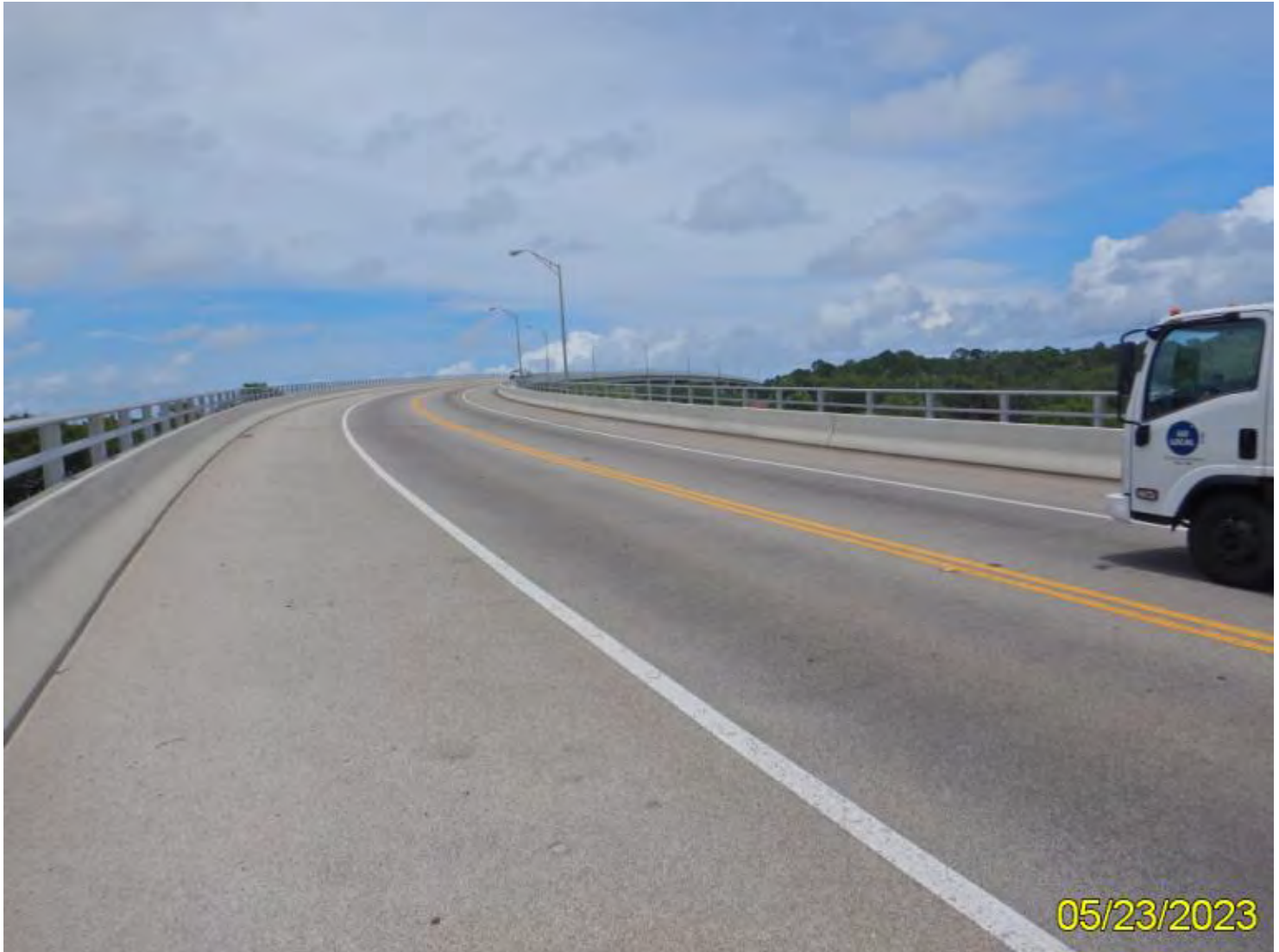
Photo 29 - Elements 331 Re Conc Bridge Railing and 333 Other Bridge Railing
