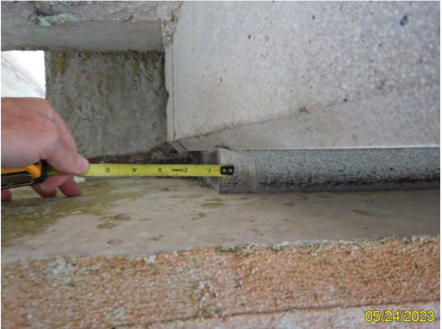
Photo 26 - Element 310 Elastomeric Bearing
