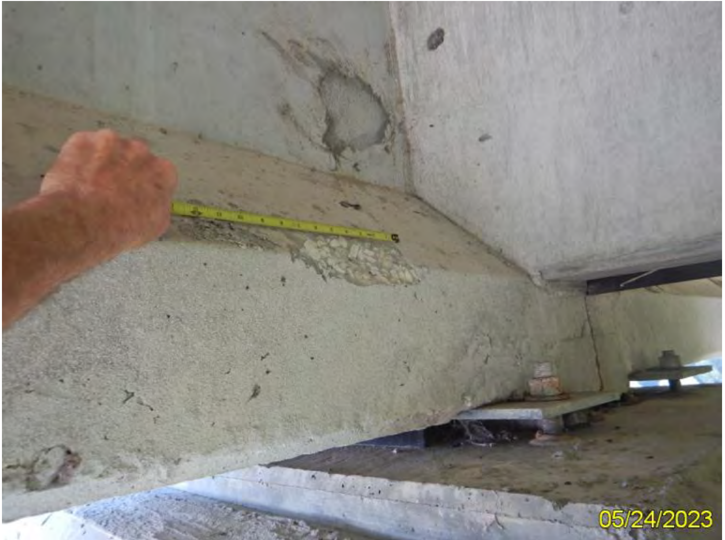
Photo 28 - Element 109 Pre Opn Conc Girder/Beam
