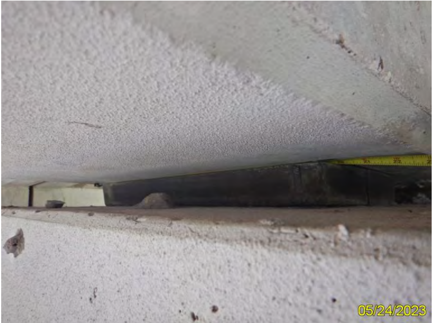
Photo 25 - Element 310 Elastomeric Bearing
