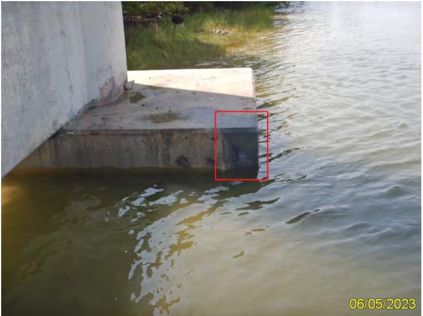
Photo 18 - Element 220 Re Conc Pile Cap/Ftg
