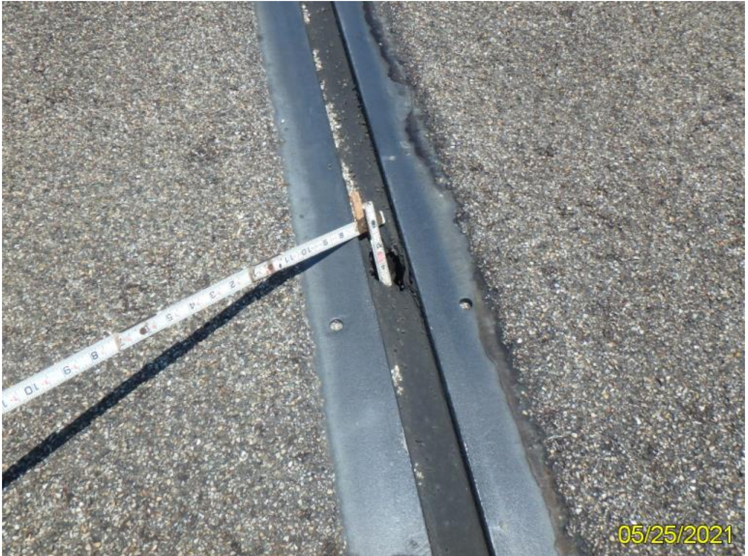
Photo 6 - Element 301 Pourable Joint Seal
