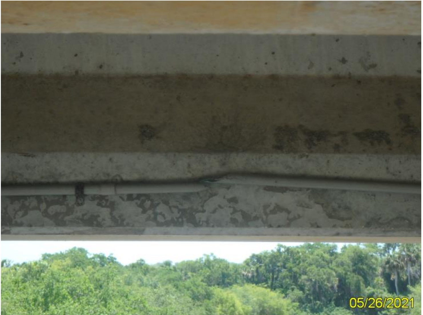
Photo 33 - Element 109 Pre Opn Conc Girder/Beam
