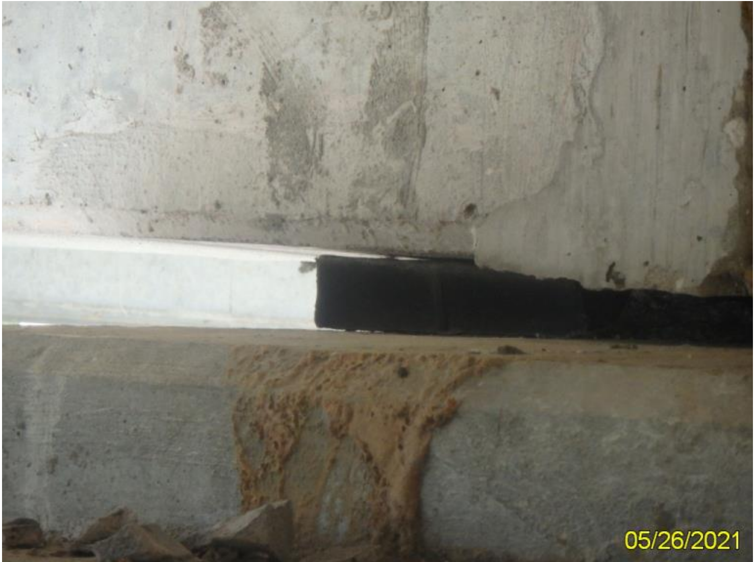
Photo 28 - Element 310 Elastomeric Bearing
