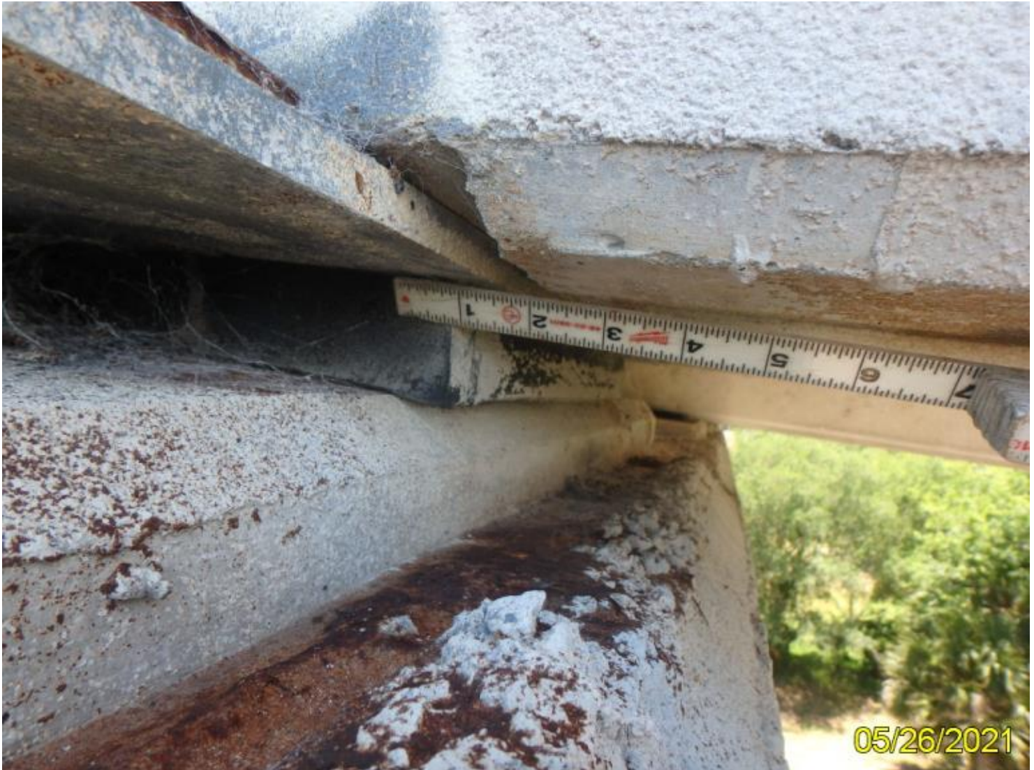
Photo 30 - Element 310 Elastomeric Bearing
