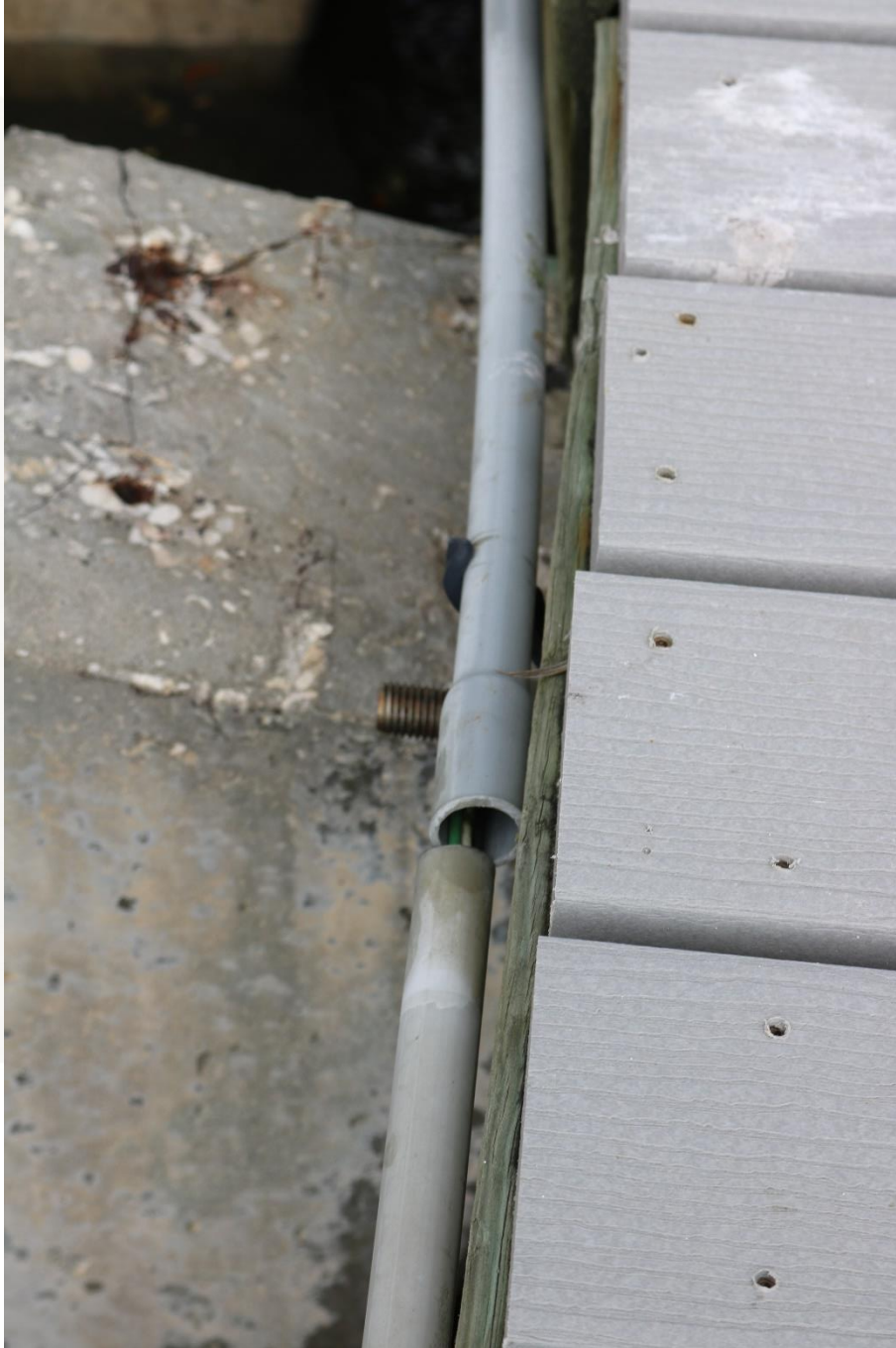
(Photo 9 - Breached Electrical Conduit)
