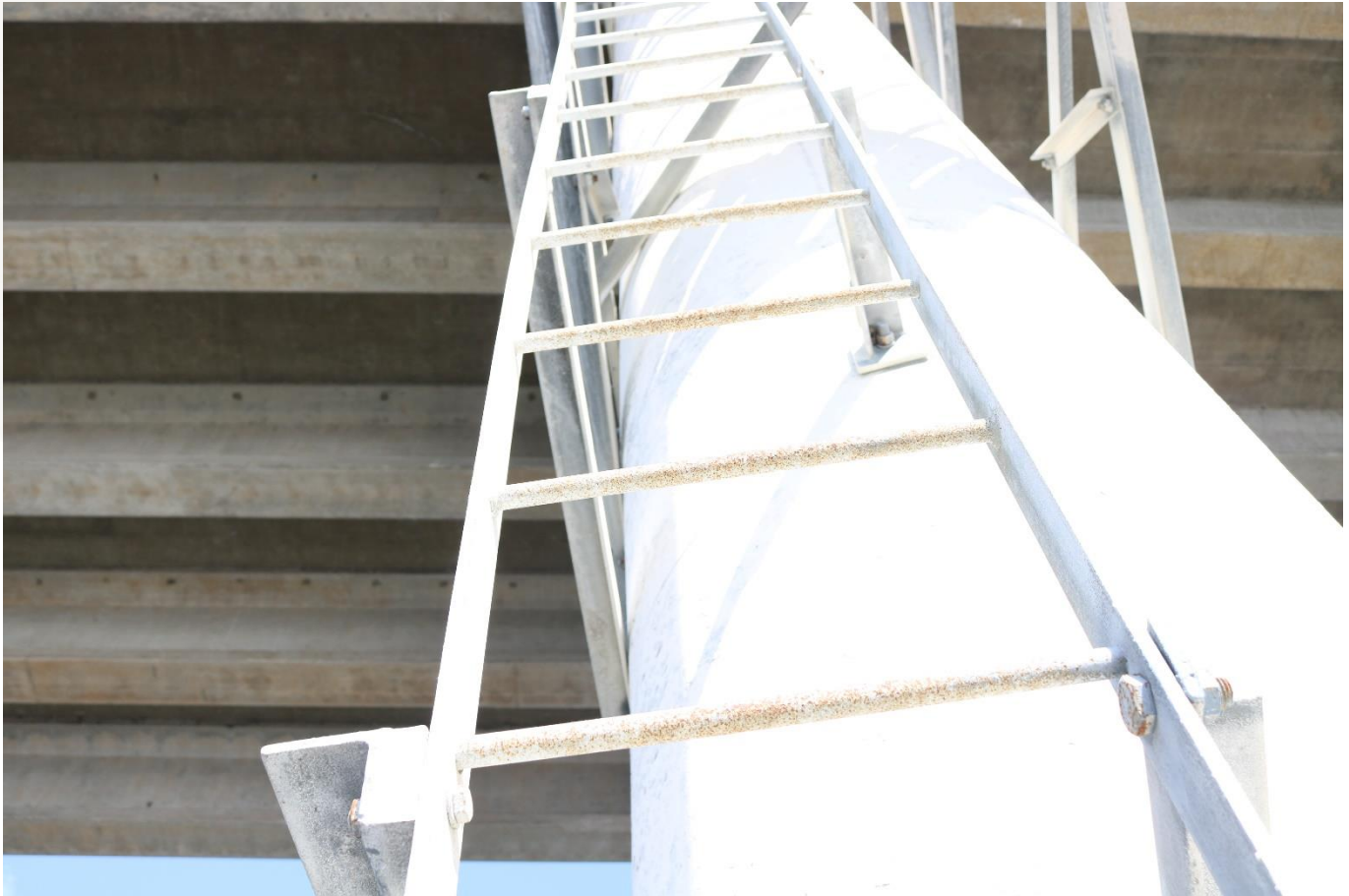
(Photo 3 - Deterioration of Hot-Dipped Galvanizing)
