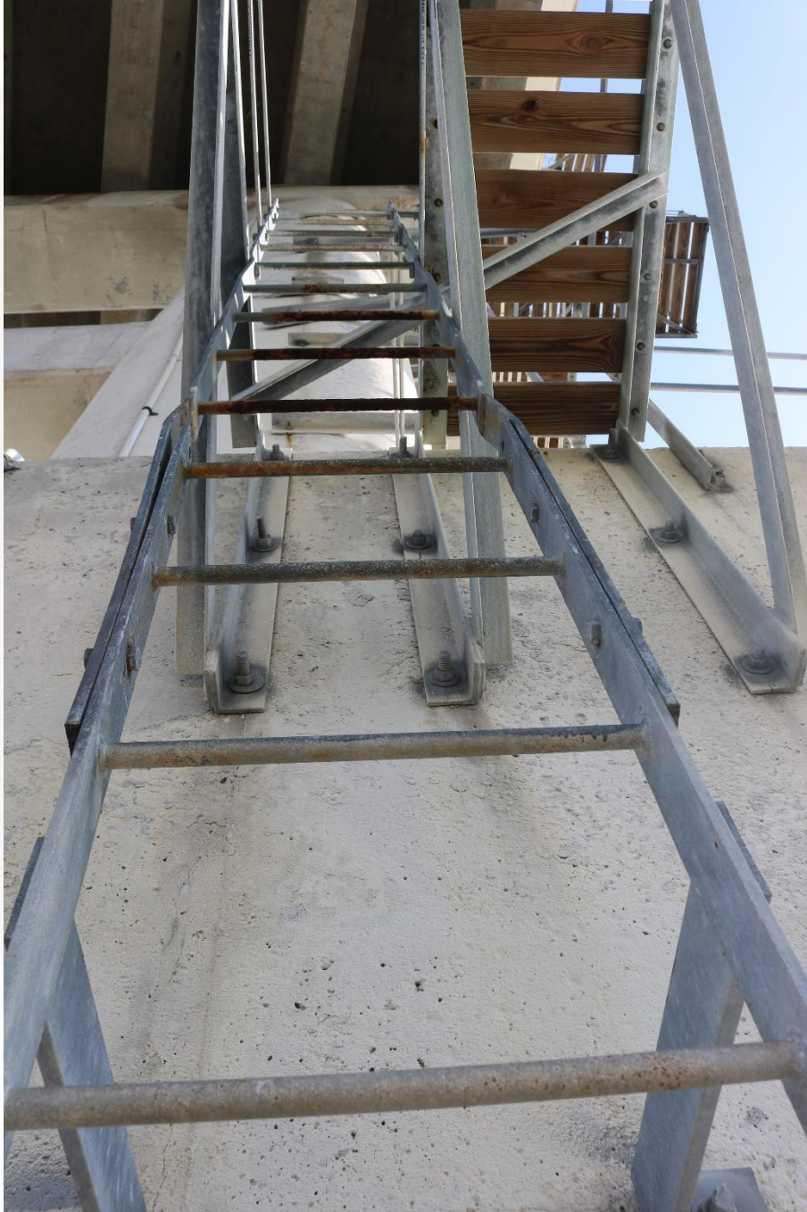
(Photo 13 - New Ladder Section Stitched in Place)
