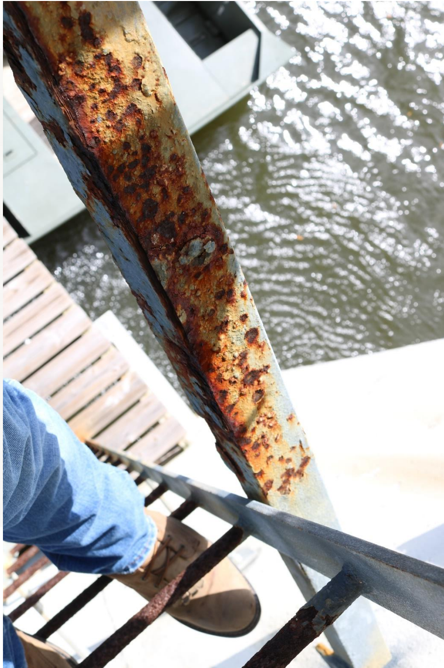
(Photo 5 - Landing Bracing Corrosion)
