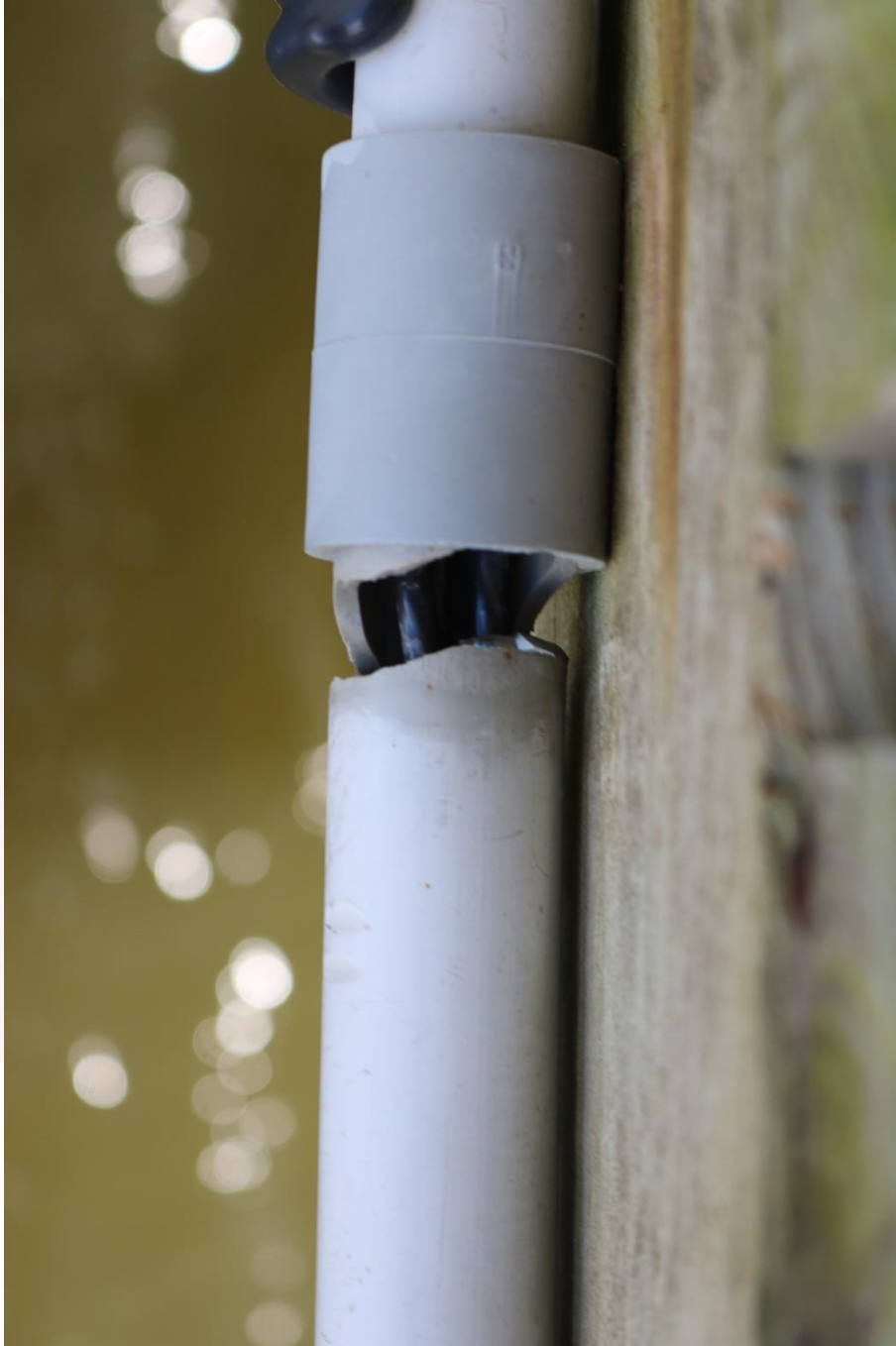
(Photo 12 - Conduit Breached Approximately at Midspan of Catwalk)
