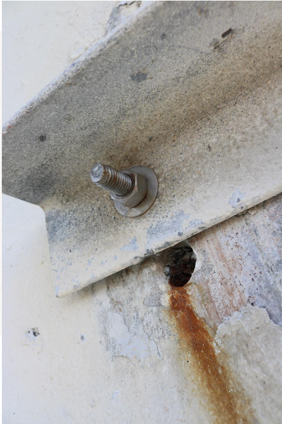
(Photo 11 - Smaller Diameter Anchors)
